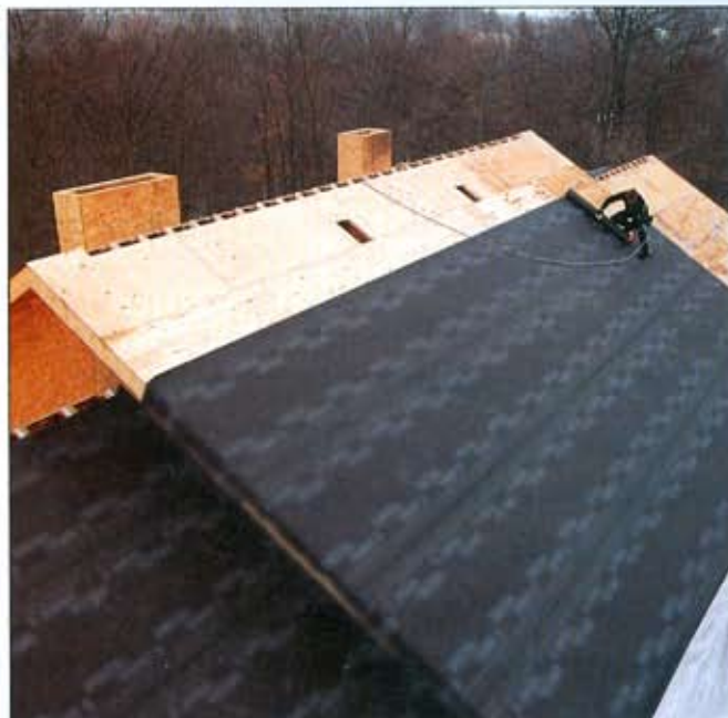
An underlayment with good moisture management characteristics is critical for a long-lasting roof, especially in cold climates.
